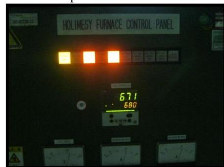
Gambar 4.a. Temperatur aluminium cair cavity yI
